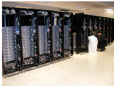
Installation des CCRT Systems
